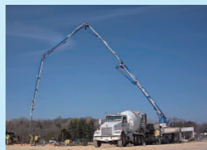
Concrete Pump Truck
