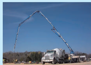
Concrete Pump Truck
